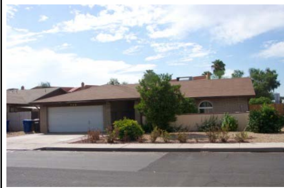
Men's Advanced Facility Main cross streets 8th Avenue & Dobson—Mesa
